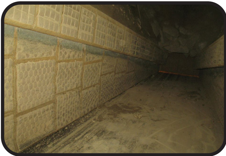
Looking toward the tail of the Loading Shoe. Top left is the engineered ceramic Deadbed Bar that protects the tapered floor of the Shoe.
