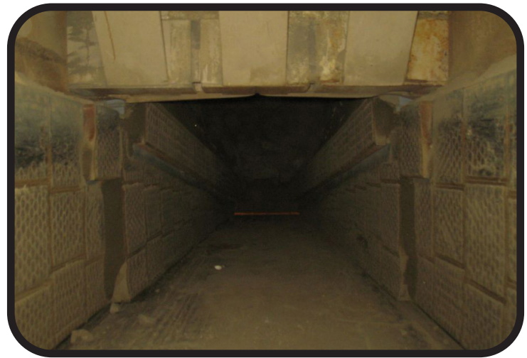
Internal Loading Shoe is fitted with ceramic liners on the Feeder Walls. Strike-off bar is overhead.
