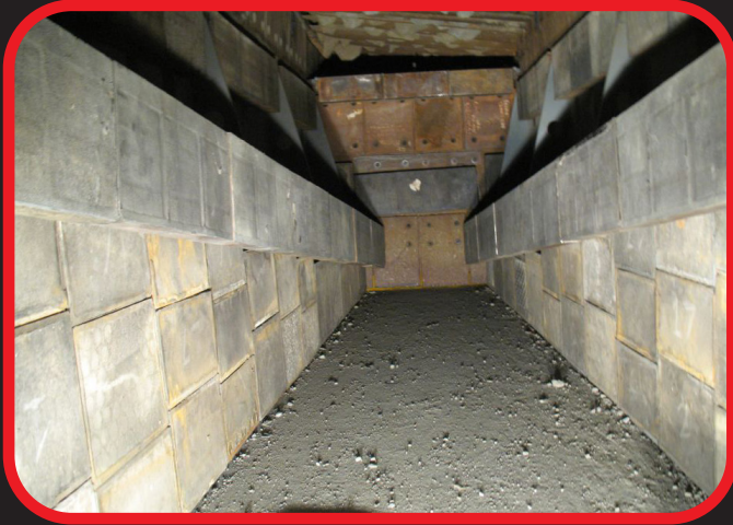
Completion of Installation
